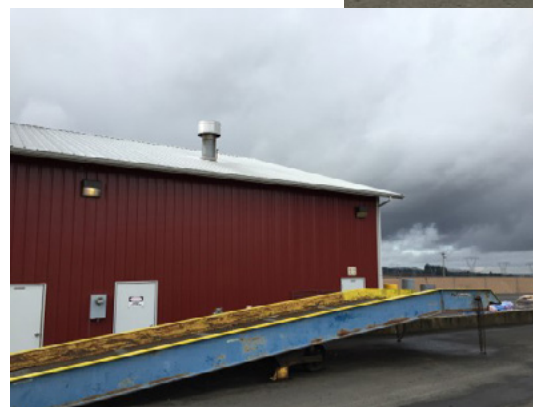
The portable ramp used to load and unload delivery trucks.
